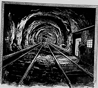
Fig. 22.—The moined Tunnel lit by Glow Lamps, after the plan of the West Construction Company.
